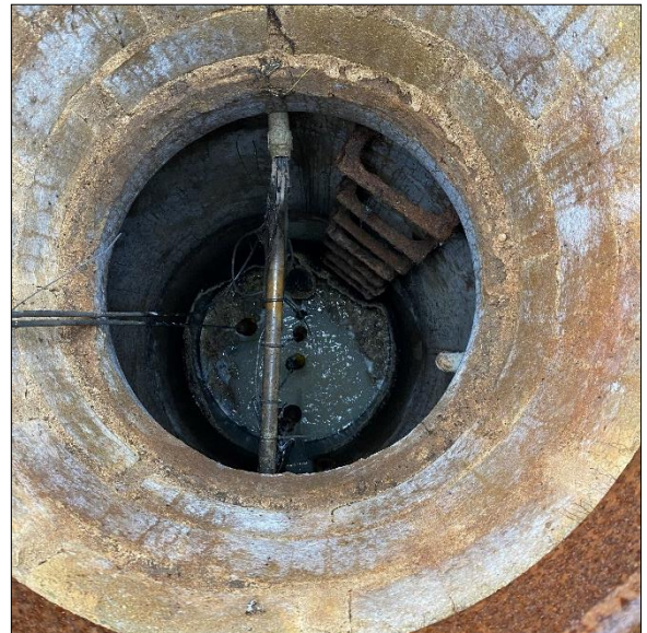
Figure 2 – Highway Lift Station Wet Well
